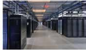
HOT AISLE CONTAINMENT
