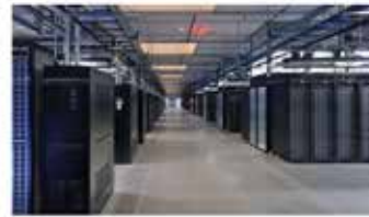
HOT AISLE CONTAINMENT
