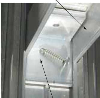
EAM-555-NC Notched Angle attached to A-50 Channel with self-drilling screw
