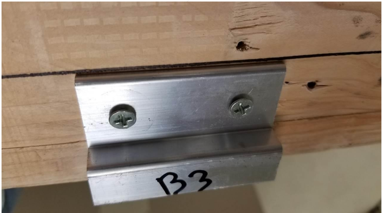
Figure 2. 2.5" clip installation (typical)
