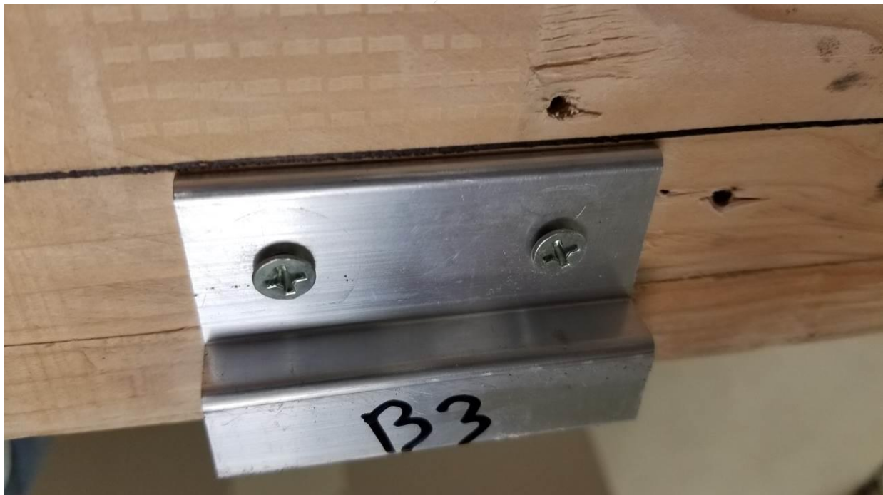
Figure 2. 2.5" clip installation (typical)
